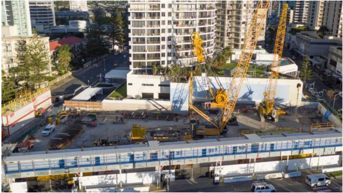
The construction site where the tower will rise Photo: Supplied
